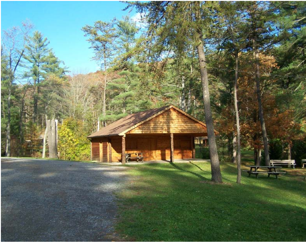
Quarter Master Building
